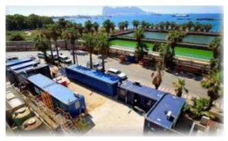
In preparation for the Maersk marine trial, a 40 tonne per hour MSAR® production system was installed at the Cepsa's 240,000 barrel per day refinery at San Roque in Spain. The equipment commissioning, fuel production and quality control activities were all undertaken by Quadrise. The plant was operational within 9 months from contract signature. Some 7,000 tonnes of MSAR® were produced and subsequently consumed by the Maersk Seago Istanbul during around 1,500
