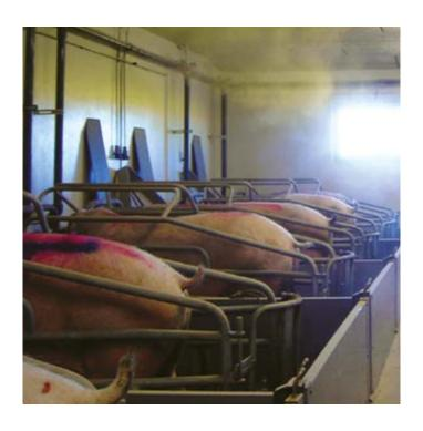
1 Illustrates Hydor Agri-Jet units mounted in the roof with inlets positioned along the two side walls. Misting nozzles are positioned internally above each inlet.
