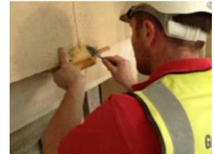
specialist restoration repair mortar (4 colours used to match stone colour).
