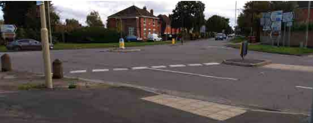
Z4.2.1 Winchester Road roundabout
