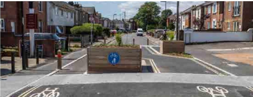
Point closure – SCN 1 Western Cycle Freeway, Southampton
