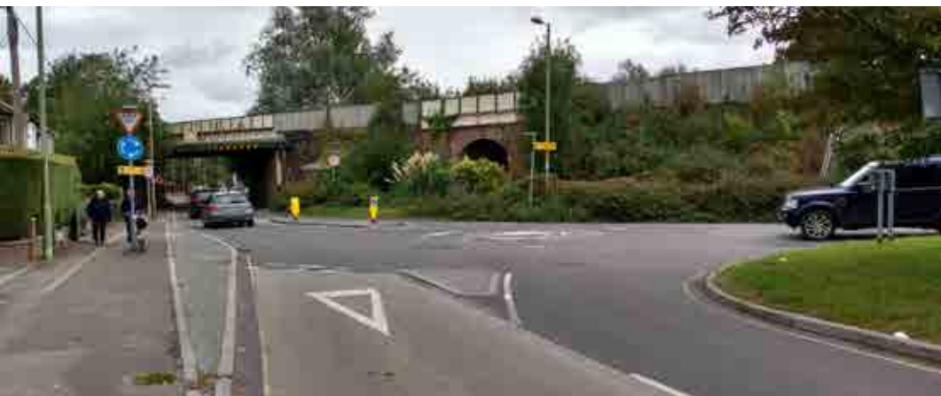
282.2.3 Greatbridge Road Roundabout
