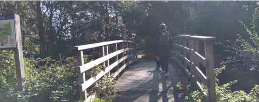
281.2.2 Withy Close canal bridge
