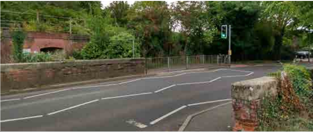
282.2.4 A3057 Train Track Underpass
