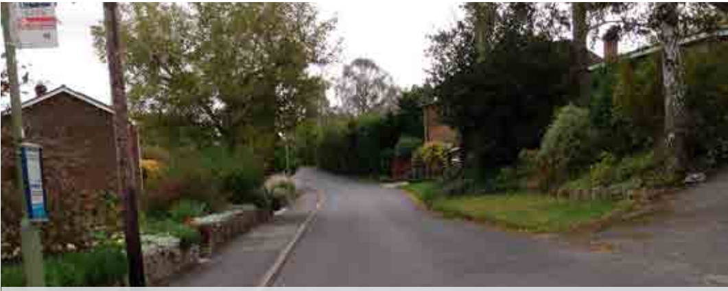
282.3.5 Richmond Lane at Brook Way Junction
