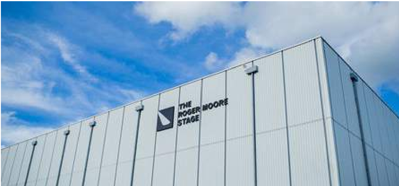
Fig 4.11: The Roger Moore Stage, Pinewood Studios
