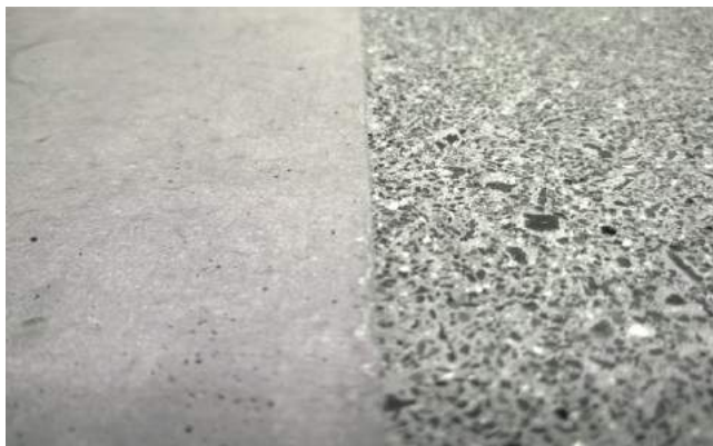
Fig 4.7: Etched concrete finish
