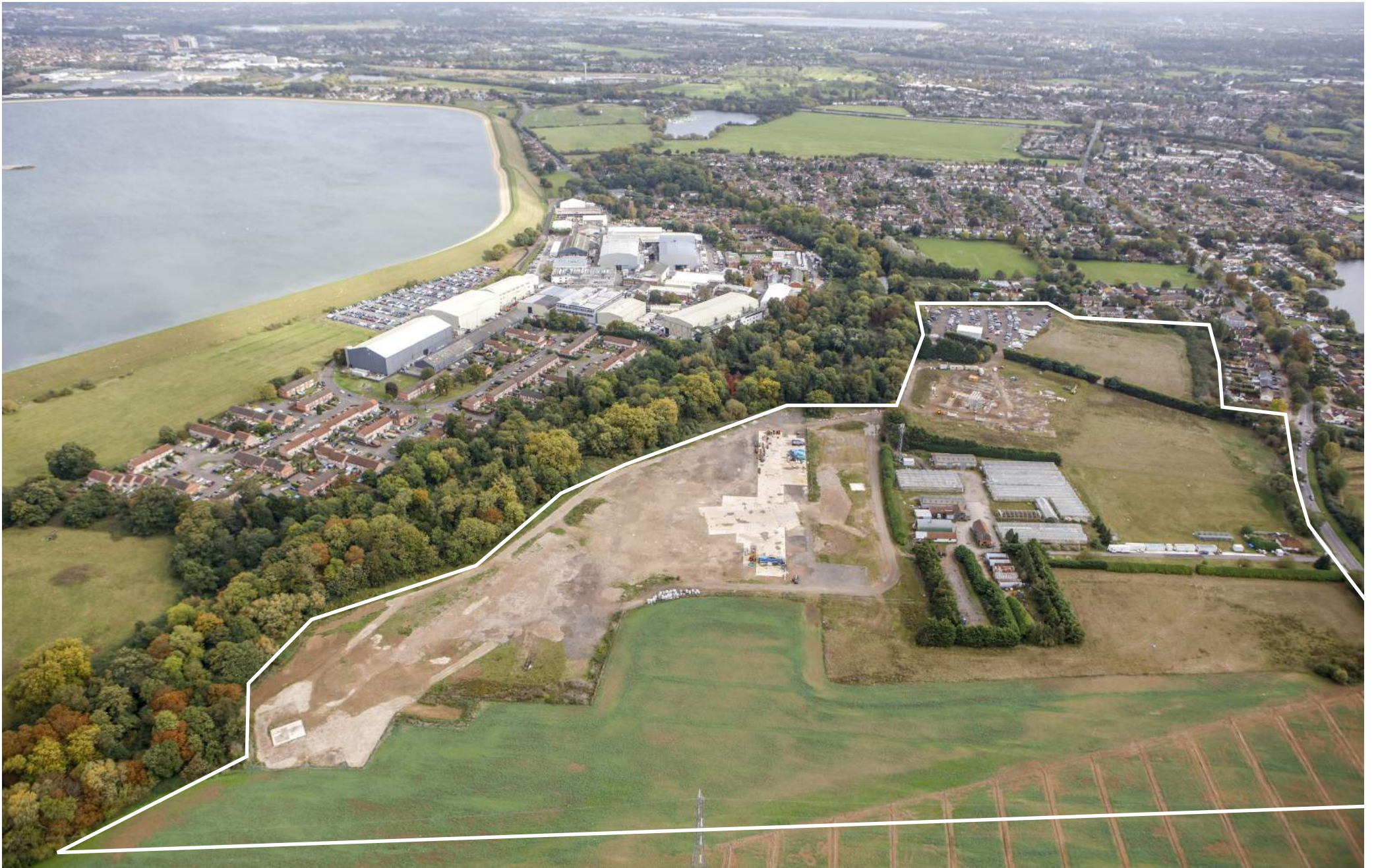
Fig 2.9: Aerial view from the west
