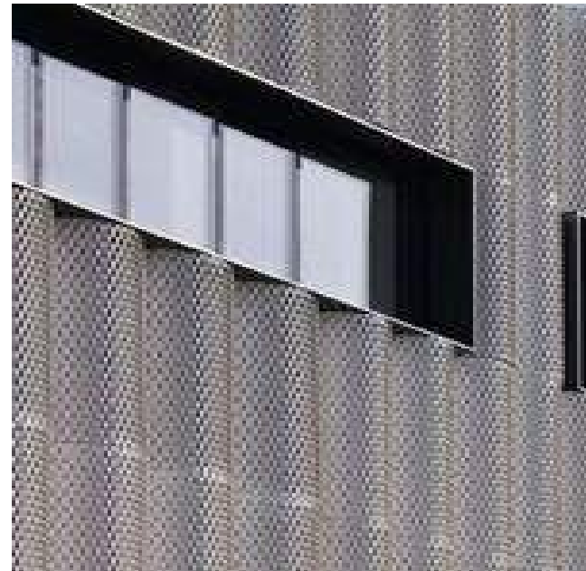
Fig 5.8: Profiled cladding with opening surrounds
