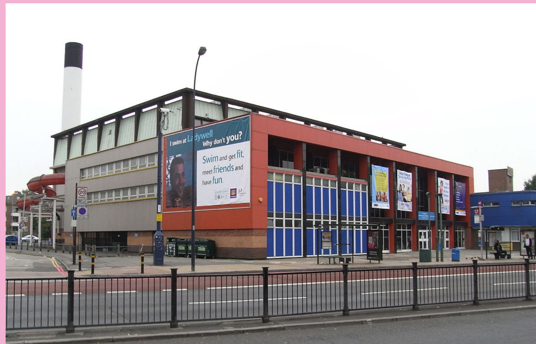
Former Ladywell Leisure Centre
