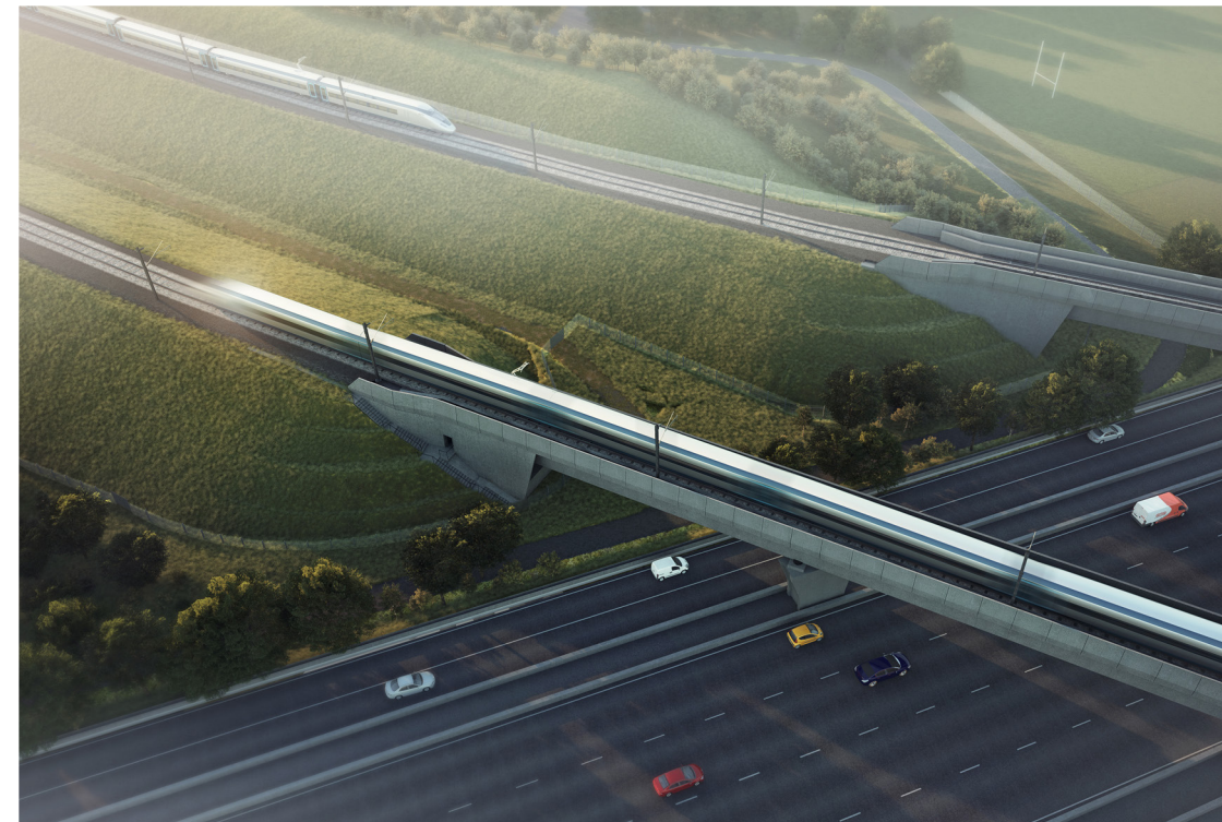
View of the abutment next to M42 motorway 10 years post-construction
