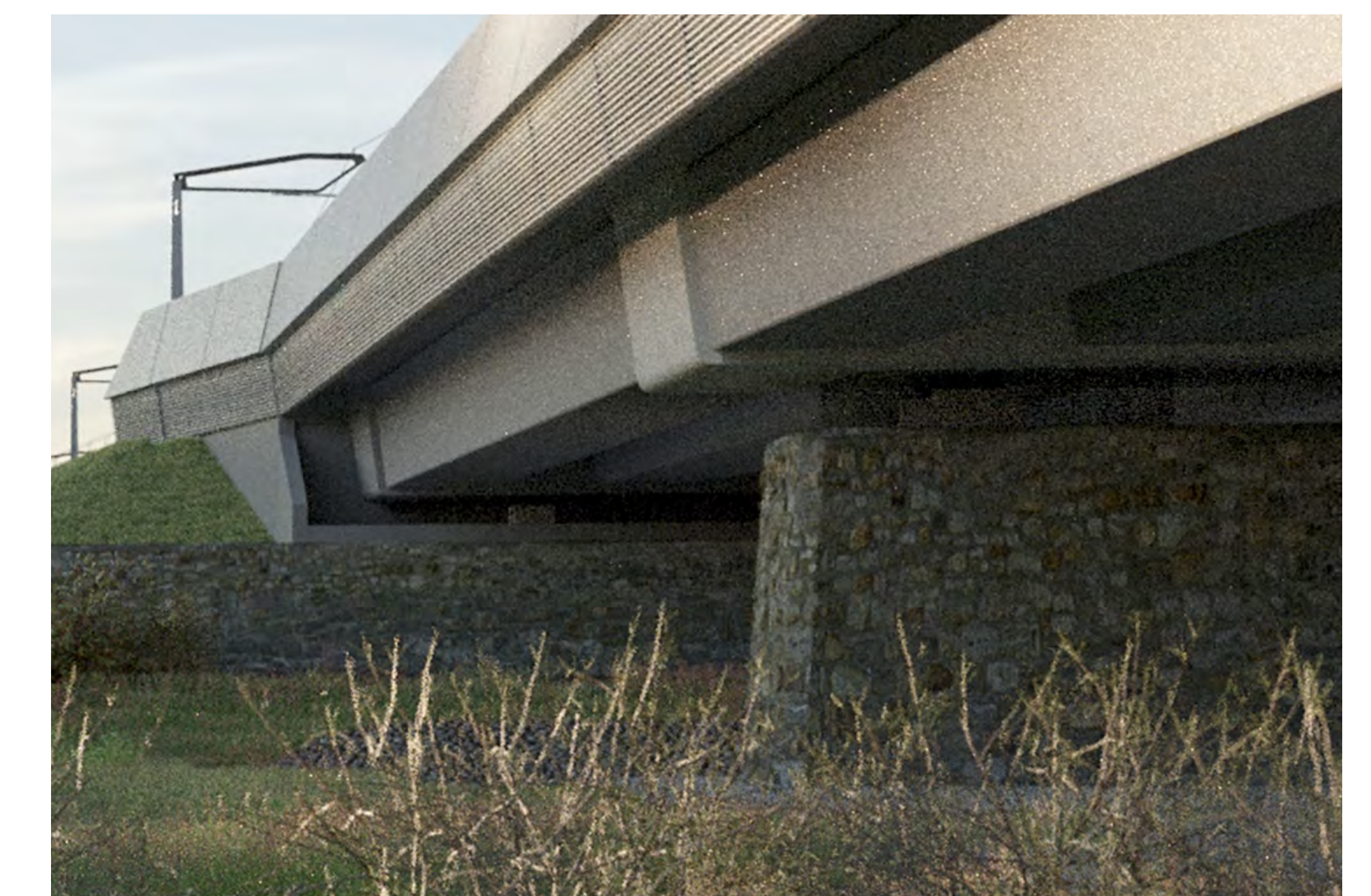
An artist's impression of the Oxford Canal Viaduct with the masonry leaf finish (Option B)
