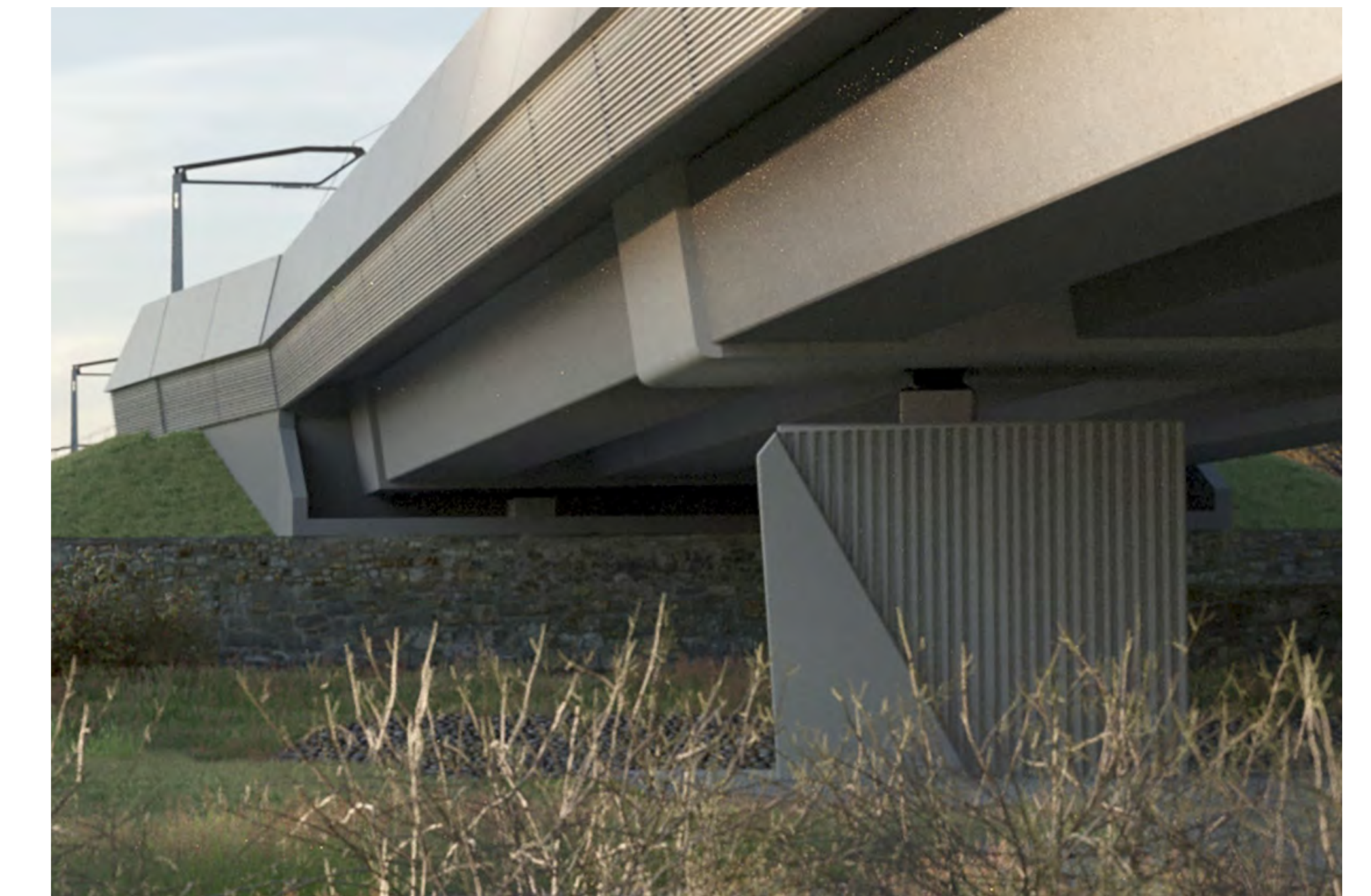
An artist's impression of the Oxford Canal Viaduct with the smooth concrete finish (Option A)
