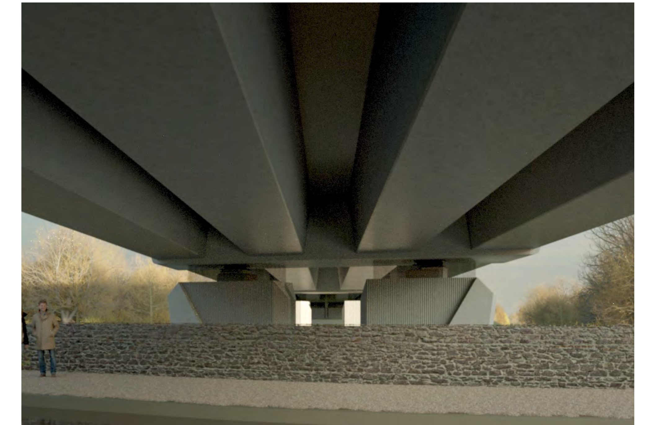
An artist's impression of the underside of the viaduct with a smooth concrete finish on the piers (Option A)
