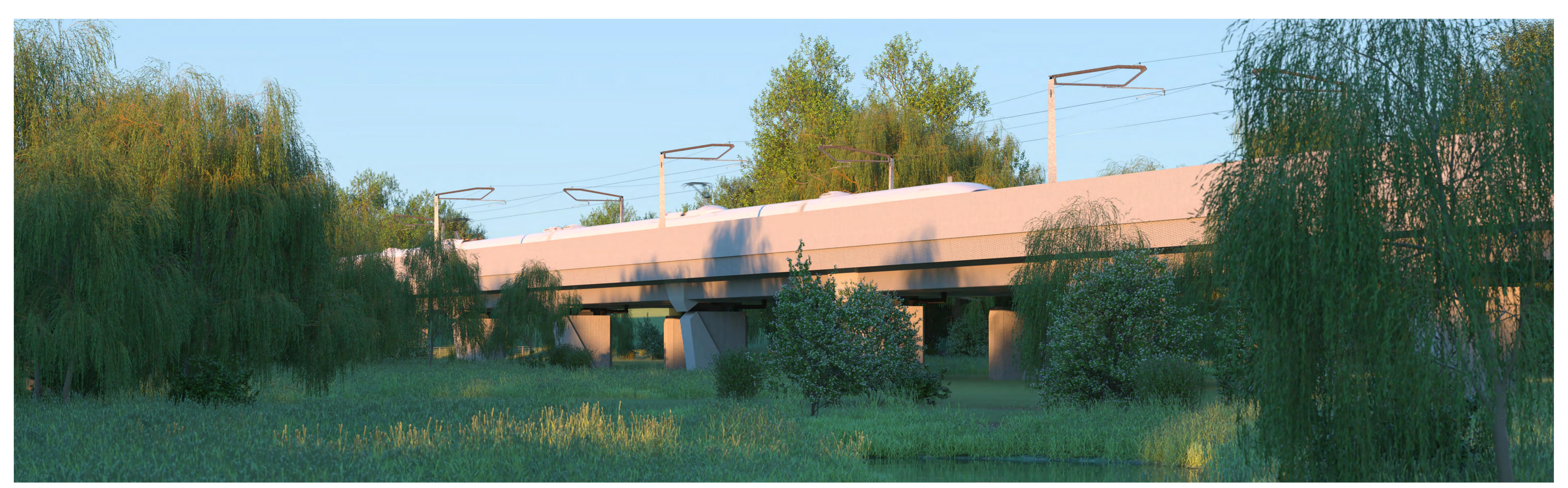
An artist's impression of the Edgcote viaduct in 10 to 15 years time, showing how the landscape will aid in masking the viaduct and the Overhead Catenary System (OCS) on top of the deck
