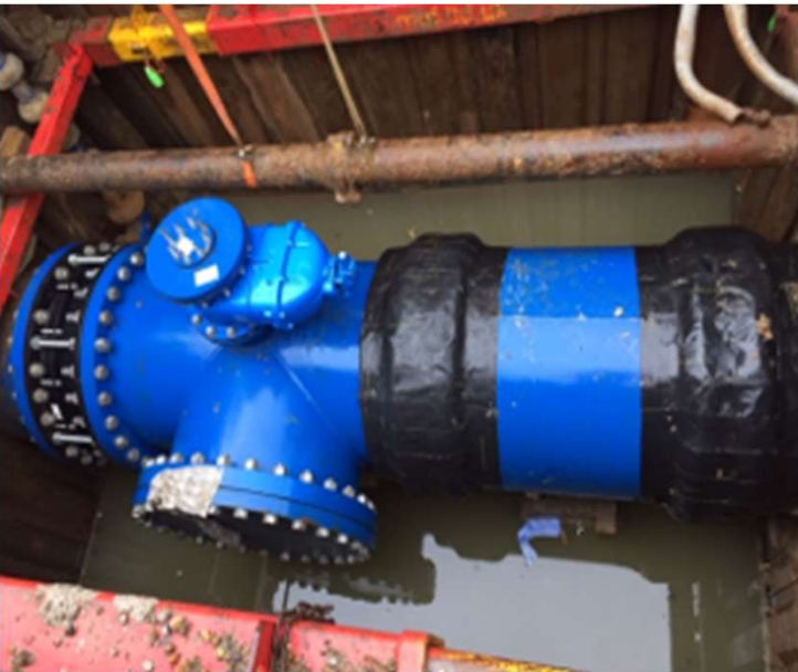
New connection in PVE on the existing 42" water main.
