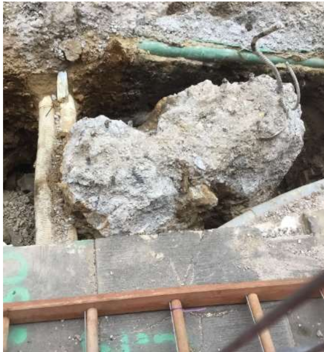
Old concrete piles that were investigated with LB Camden
