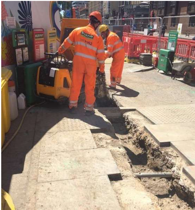
Tracked barrow used to transport material due to congested utilities
