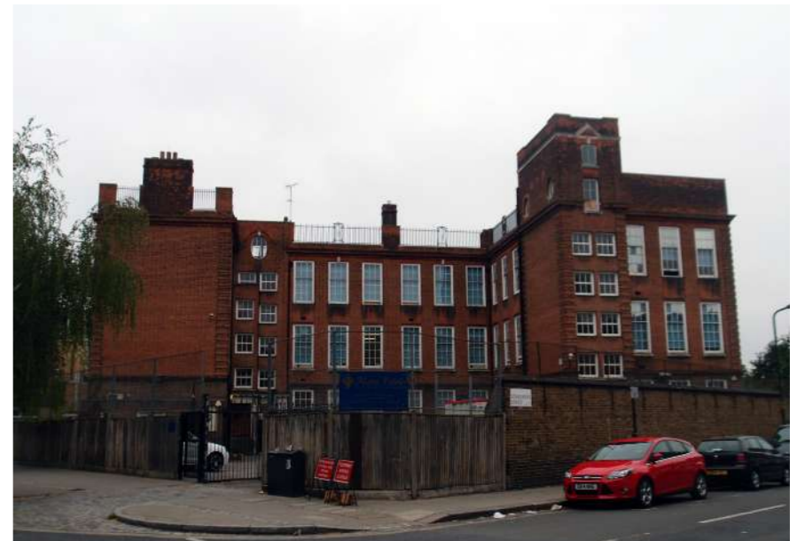
View of the main entrance with parking to the former Maria Fidelis School
