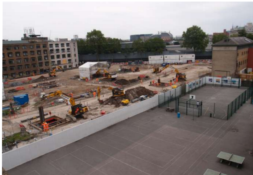
View from roof of the former Maria Fidelis School
