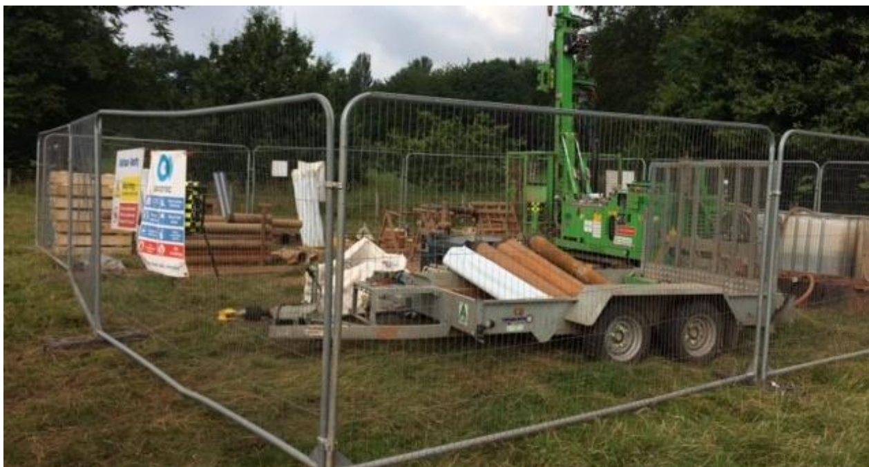
Example of trial boring that make up part of the ground investigation work
