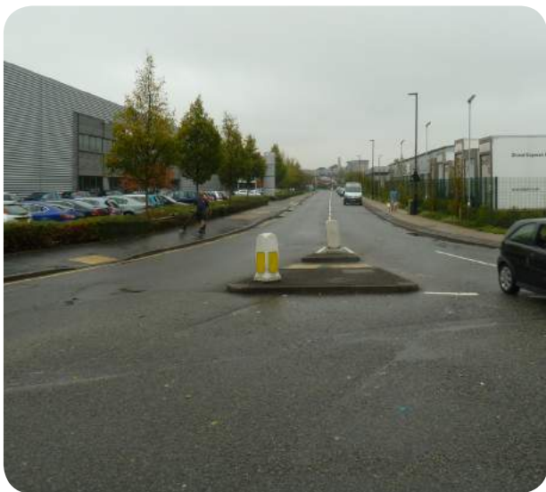
Irregular frontages in industrial areas
