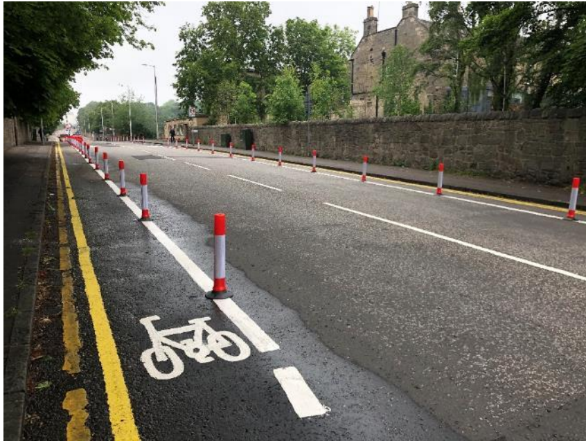
Figure 7: Example of a traffic cylinder delineator posts layout to temporarily define space for cycling
