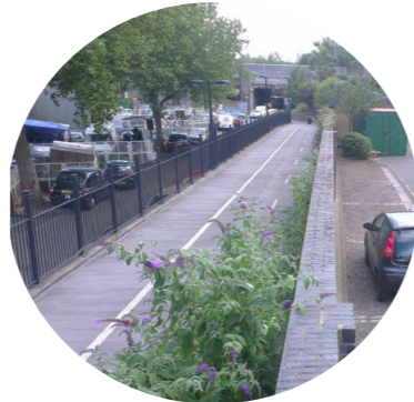
Level changes and poor legibility around the area
