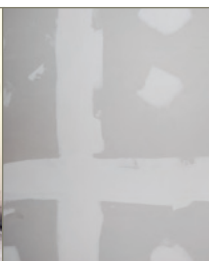
Spackled Repairs
