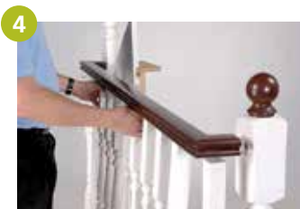
Once all the fittings have been removed, the section of assembled balustrade is simply lifted off.
