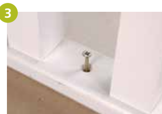
Unscrew the floor rail.
