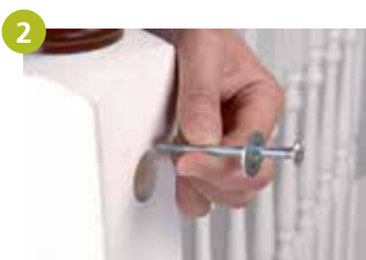
Unscrew and remove the bolt holding the handrail and keep safely.
