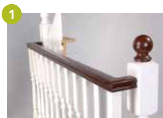
The balustrade fully assembled.
