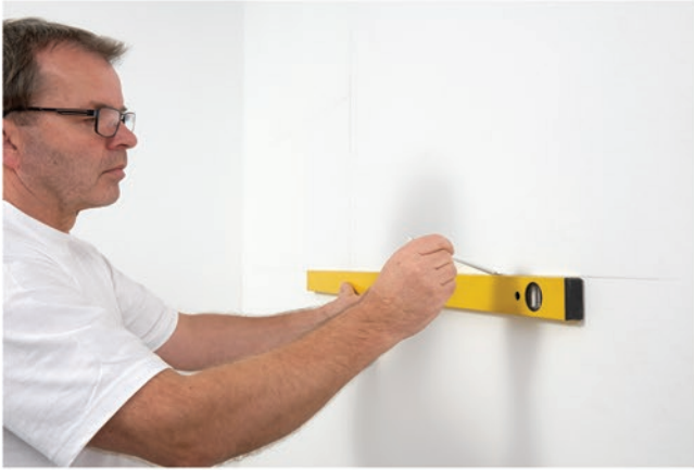
1. Measure out the wall and define the position of the panels.
