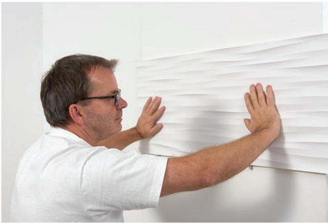
3. Position the panel (spacers recommended for Designer Panels 1 & 2).
