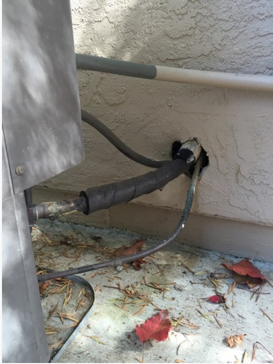
Refrigerant lines penetrating the stucco, the open gap, should be sealed.
